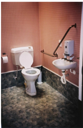
An accessible toilet is shown above. Notice the door width, high toilet, placement of rails and spacious cubicle for easy transfers.
